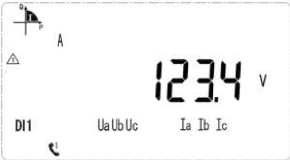
Voltage on A phase is 123.4V
